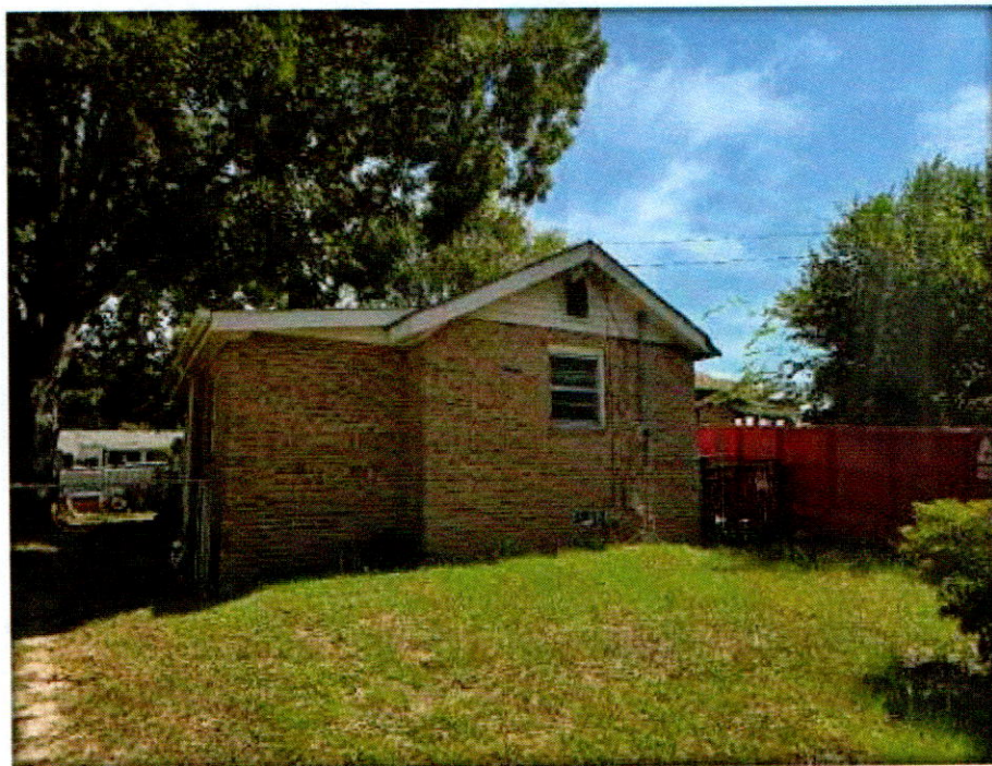
Photographs Blight Removal Project 1937 Henry Street, Fayetteville, NC 28306
